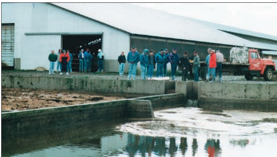
Fig. 6. Fixed passive manure separation with two cells.
